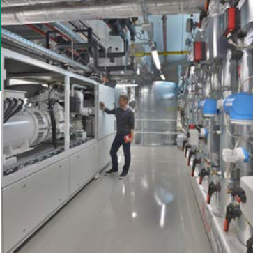
In the basement of Fraunhofer IISB: Cogeneration plant and thermal storage.
